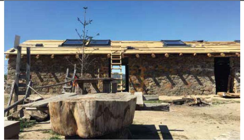
Figure 3.10: A photograph from Yayla House Construction Site
