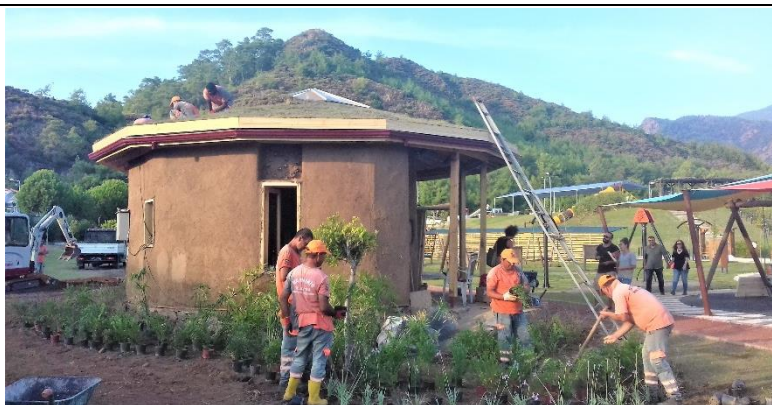
Figure 3.22: A photograph from the construction site of EcoDemo House.
